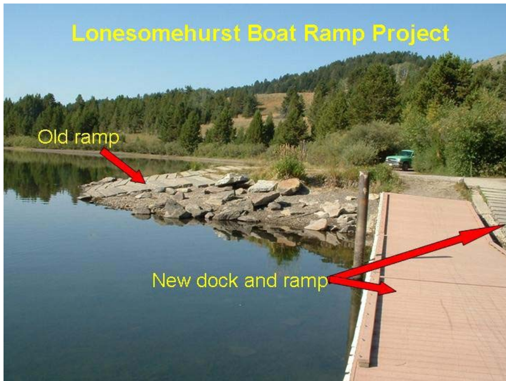
Old step ramp in relation to newer shallow ramp
