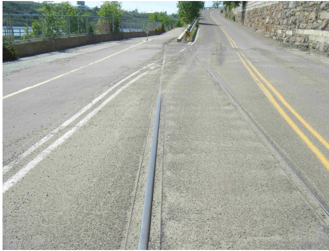
Photo of Railroad Tracks in Access Road
