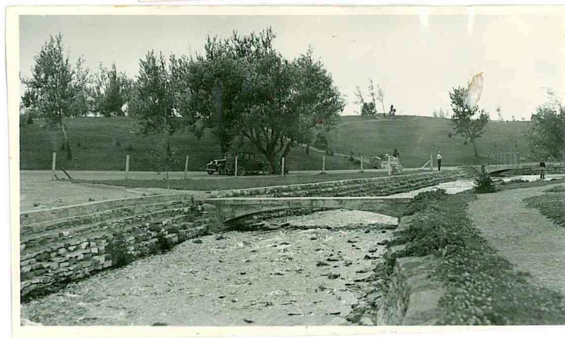
Historic Photo of Roe River Bridge (Note Depth of Roe River and Abutments out of the Water)
