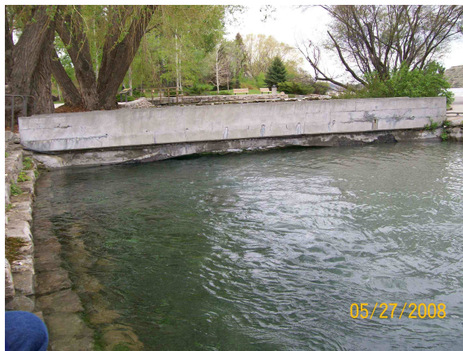
Photo of Seasonal High Water Conditions on Roe River Bridge taken 5/27/08
